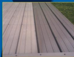
One Kynar 500 panel was included and installed on a Si-Poly project in Ohio. Note how it has retained its color after 5 years of Ohio weather.
