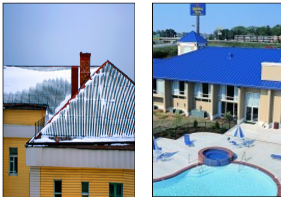
Figure 7-7 Temperature Extremes Are Normal for Any Roof
