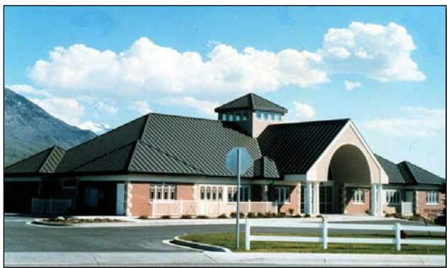
Figure 4-3 Vertical Roof Panel Installation
