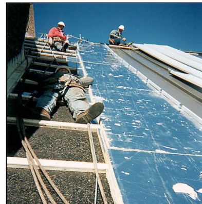
Figure 10-13 Installation of Rigid Polyiso Insulation
