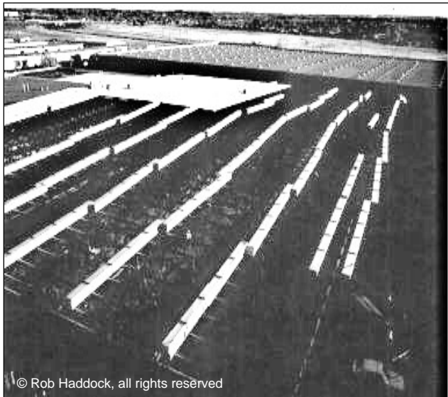
Figure 11-8 Pre-Staging Material on the Roof Has Many Advantages But Caution Must Be Used
