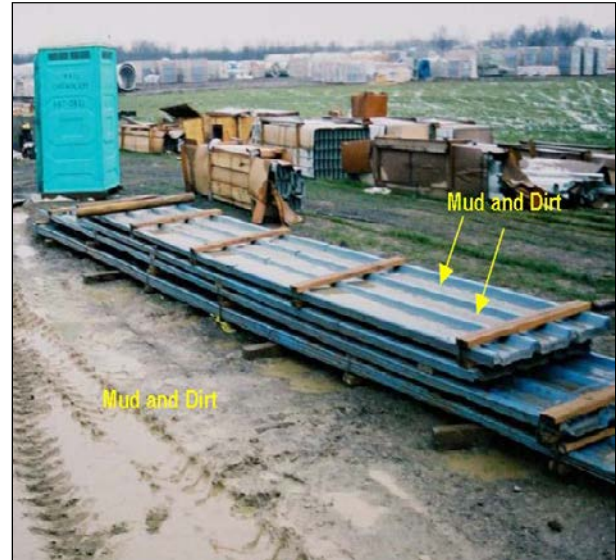
Figure 11-9 Ground Locations Are Subject To Mud Splashes
