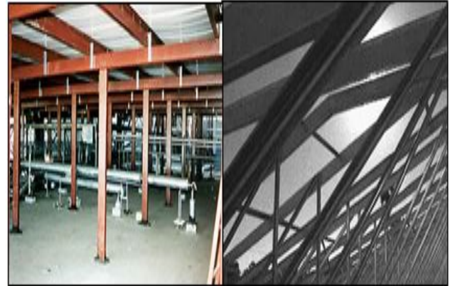
Figure 19-8 Roof Inspections Should Begin Inside the Building
