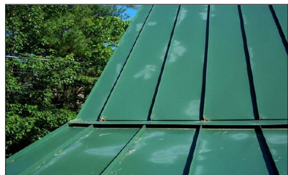
Figure 17-7 Touch-Up Paint Does Not Weather Like That of the Original Roof Panel
