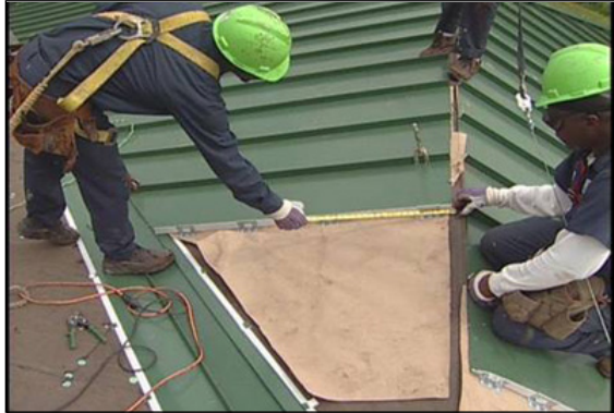
Figure 10-30 Slip Sheets Prevent Metal Roof Panels from Sticking to Underlayment, Preventing Rips and Tears
