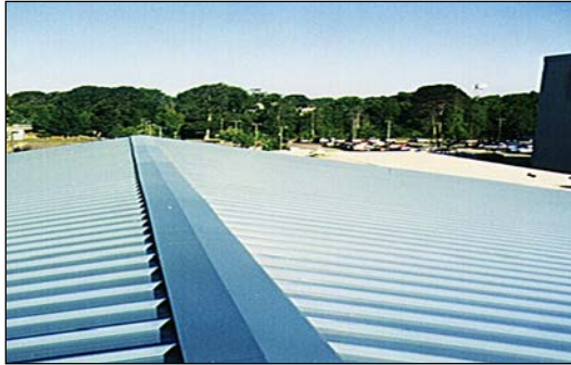
Figure 8-1 A Low-Profile Ridge Vent Blends In with the Rest of the Roof Profile
