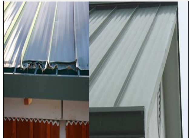
Figure 19-11 Edge and Rake Inspection
