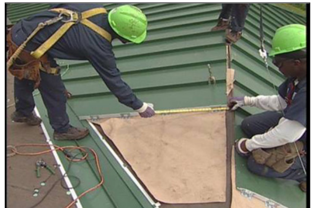
Figure 6-5 A Slip Sheet Is Often Installed Between the Underlayment and the Roof Panel.
